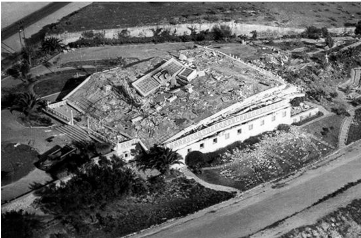
The Hotel Saada before and after 29 February 1960. Four factors – its shallowness, its intensity, its proximity to Agadir and the near-total absence of any seismic-resistant buildings – combined to maximise the earthquake's destructive force.
